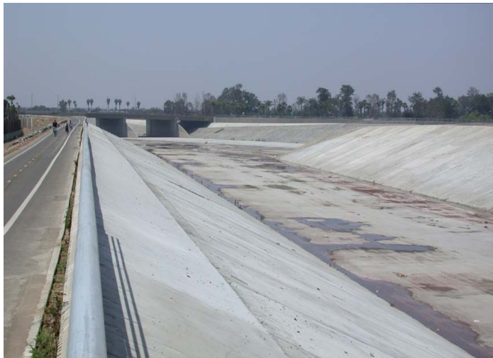
Figure 5 The Los Angeles River. Once a viable water body the river was converted into a flood conveyance channel without a base flow and with no aquatic life.
