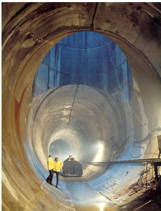
Figure 1 Deep tunnel storage in Milwaukee drilled in the dolomite rock. A longer tunnel was drilled in Chicago by a similar mining drilling machine.
