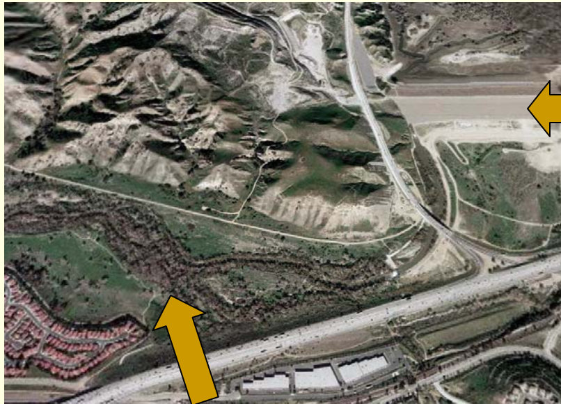
Natural Channel below Prado Dam
