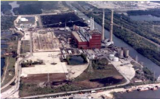
Will county power plant
