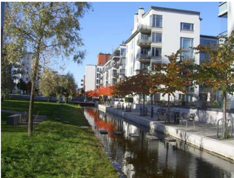
Figure 3 Hammarby Sjöstad (Stockholm) with surface drainage (Photo credit Malena Karlsson, GlashusEtt, Hammarby Sjöstad). The surface drainage collects all clean water flows (rain, groundwater, cooling).
