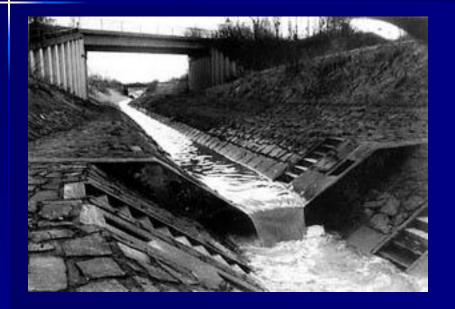
In early 1900's the Emscher River in Germany was designated and channelized solely for wastewater effluent conveyance.
