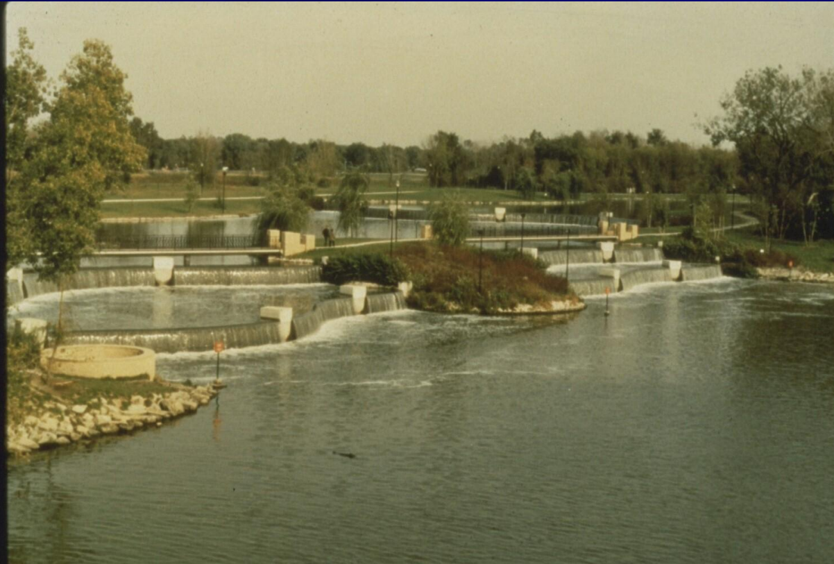
Side Elevated Pool Aeration – SEPA on Chicago waterways, water is pumped to the upper pool and cascades back while aerating (courtesy MWRD of Greater Chicago)
